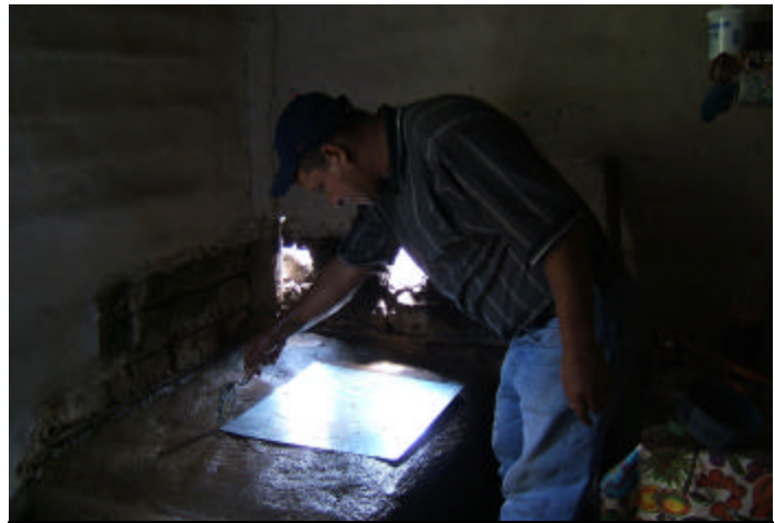
Building a Lorena stove
